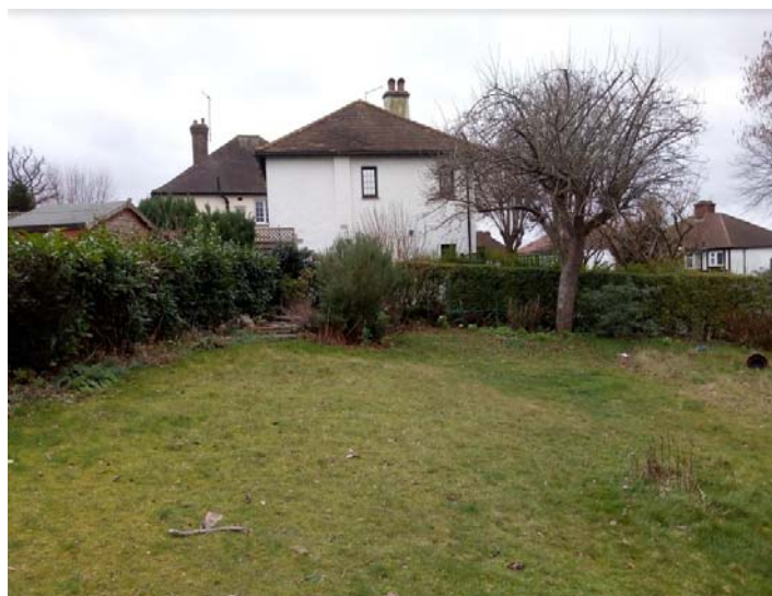
Photo 1 – Flank wall of 1 Purley Hill taken from the sites' garden.
